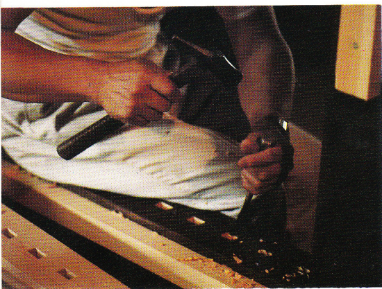
Top: Intent on his task, one of the carpenters chisels holes in a beam to support the latticed bay windows forming the shop front.
